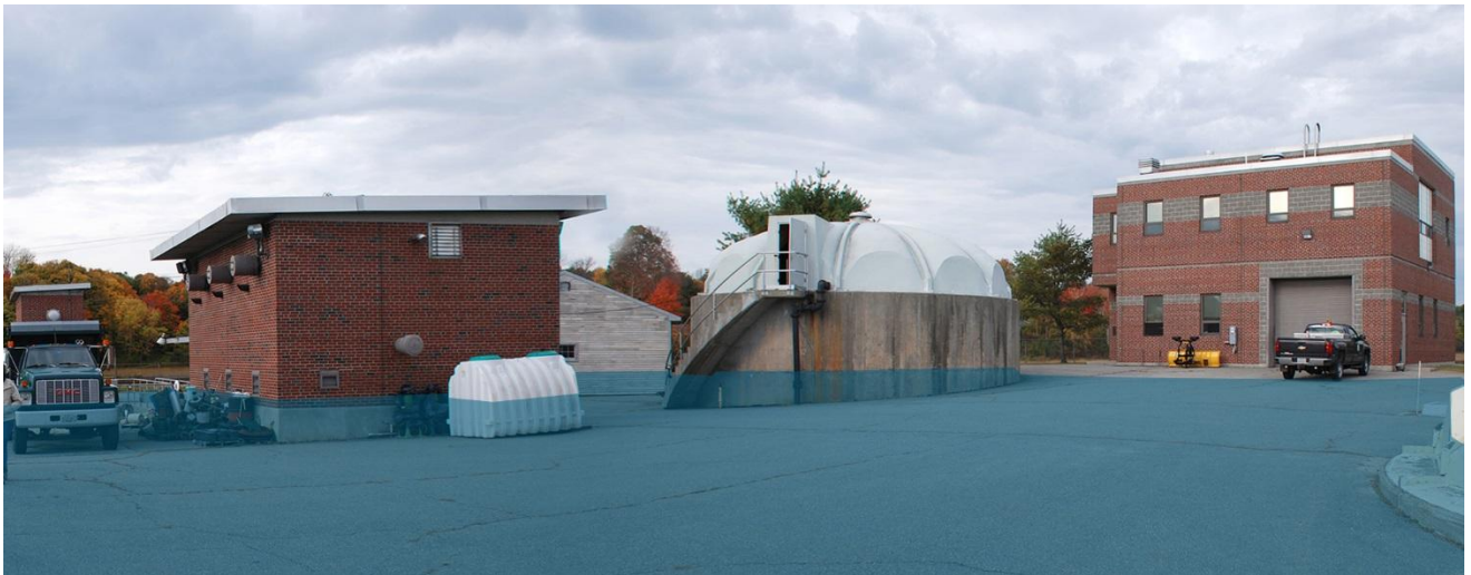
(Left to Right) Headworks Bldg, Blower Bldg, Shed, Sludge Storage, Control Bldg – BFE +3
