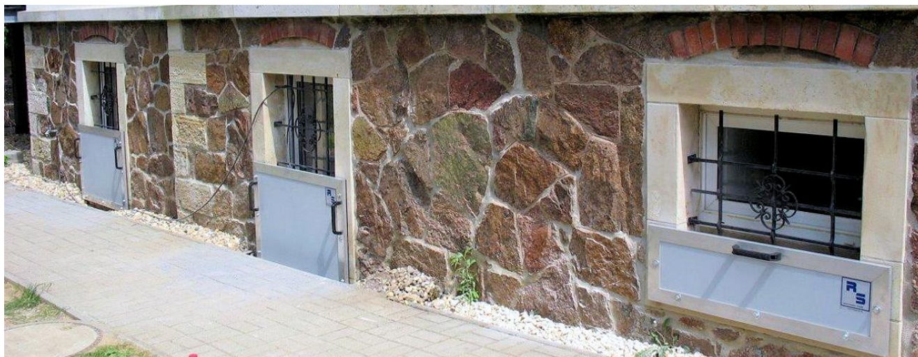
Examples of Temporary Flood Barriers for Windows (source from R S Flood Control)
