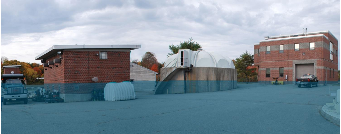
(Left to Right) Headworks Bldg, Blower Bldg, Shed, Sludge Storage, Control Bldg – BFE +6
