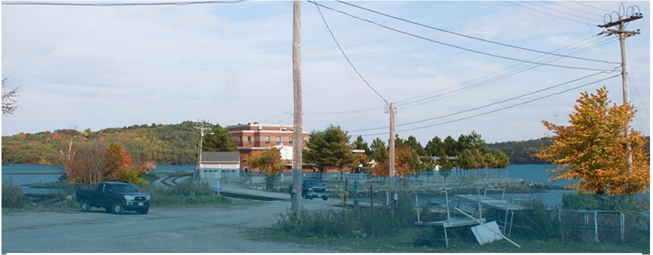
Site Approach Along Railroad Avenue Looking North Towards The WWTP – BFE +6
