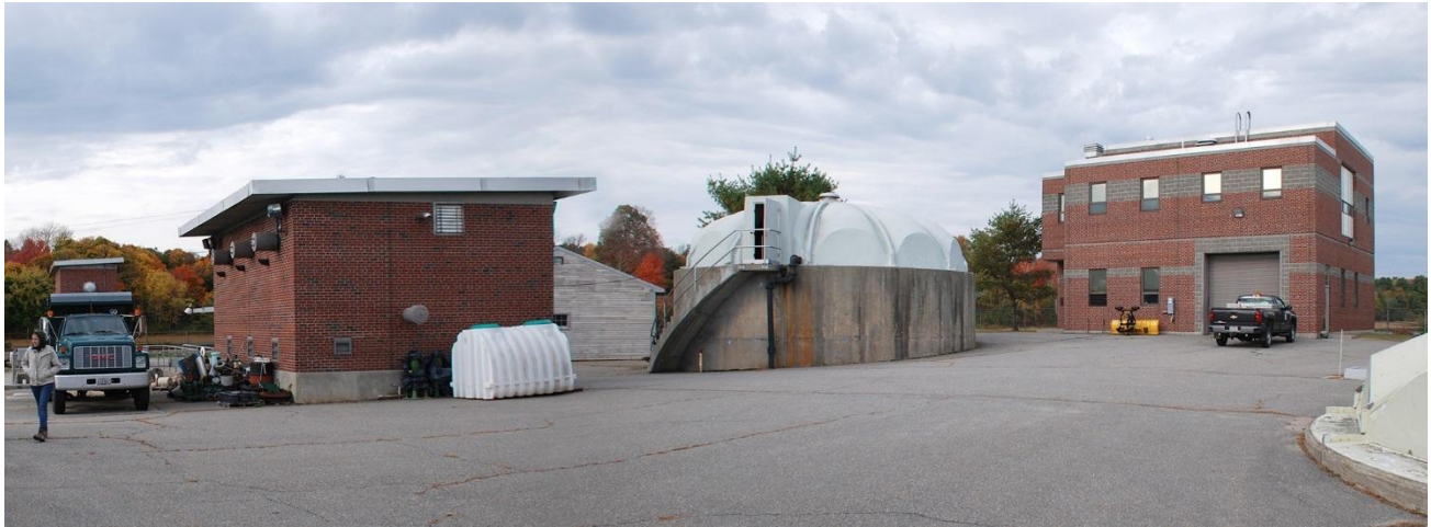
From left to right: Head works building; disinfection/ blower building; shed; sludge storage; and control building
