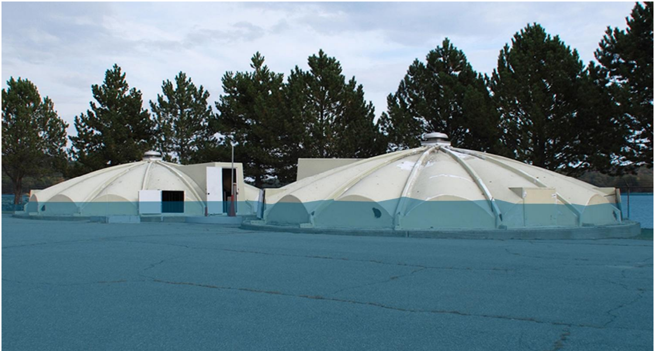
Clarifiers Looking East – BFE +4
