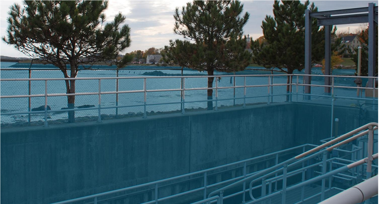
Chlorine Contact Tank Looking South – BFE +3
