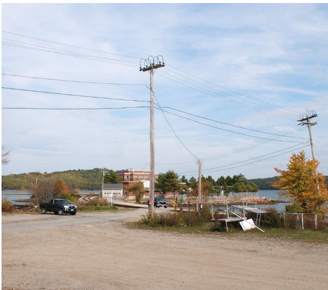
WWTP approach from Railroad Avenue
