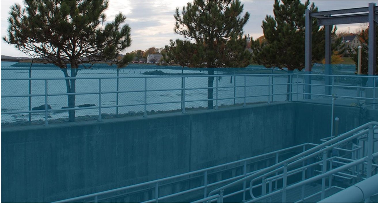
Chlorine Contact Tank Looking South – BFE +6
