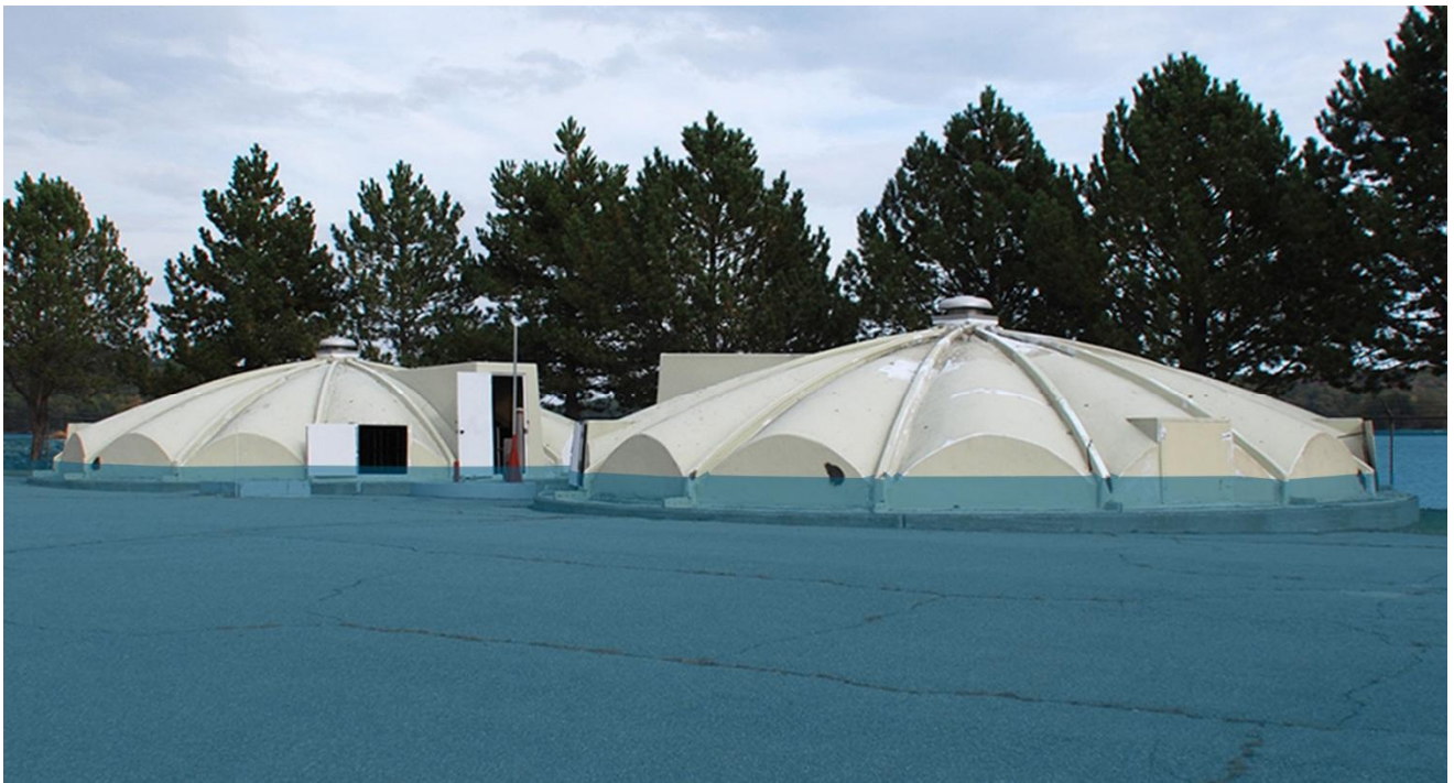
Clarifiers Looking East – BFE +3
