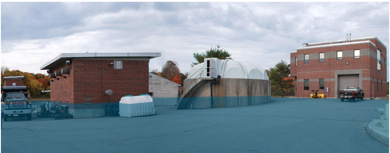
(Left to Right) Headworks Bldg, Blower Bldg, Shed, Sludge Storage, Control Bldg – BFE +4
