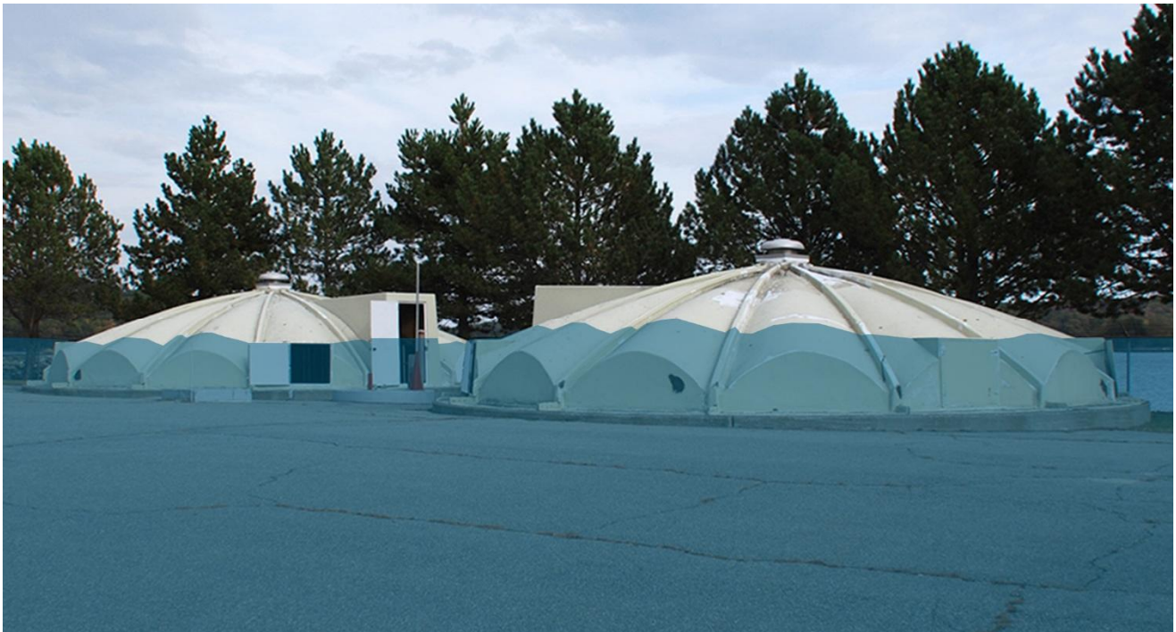
Clarifiers Looking East – BFE +6
