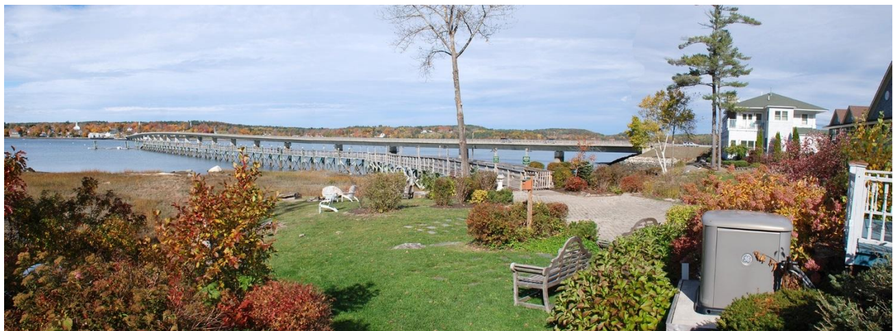
View from Edgecomb Pump Station site towards Wiscasset and across the Sheepscot River. Route 1 Bridge in the background
