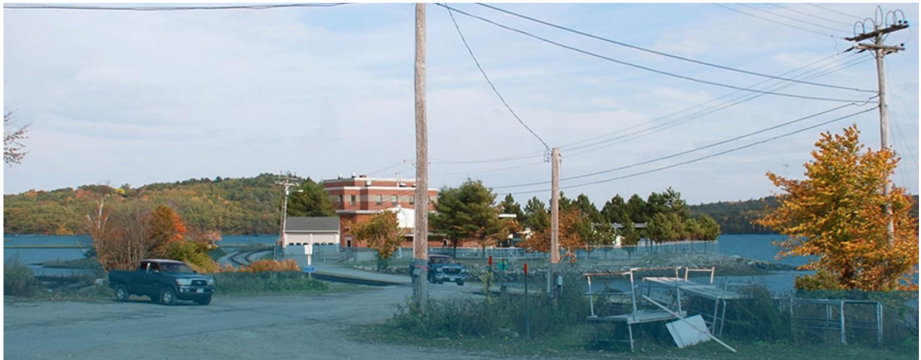
Site Approach Along Railroad Avenue Looking North Towards The WWTP – BFE +4
