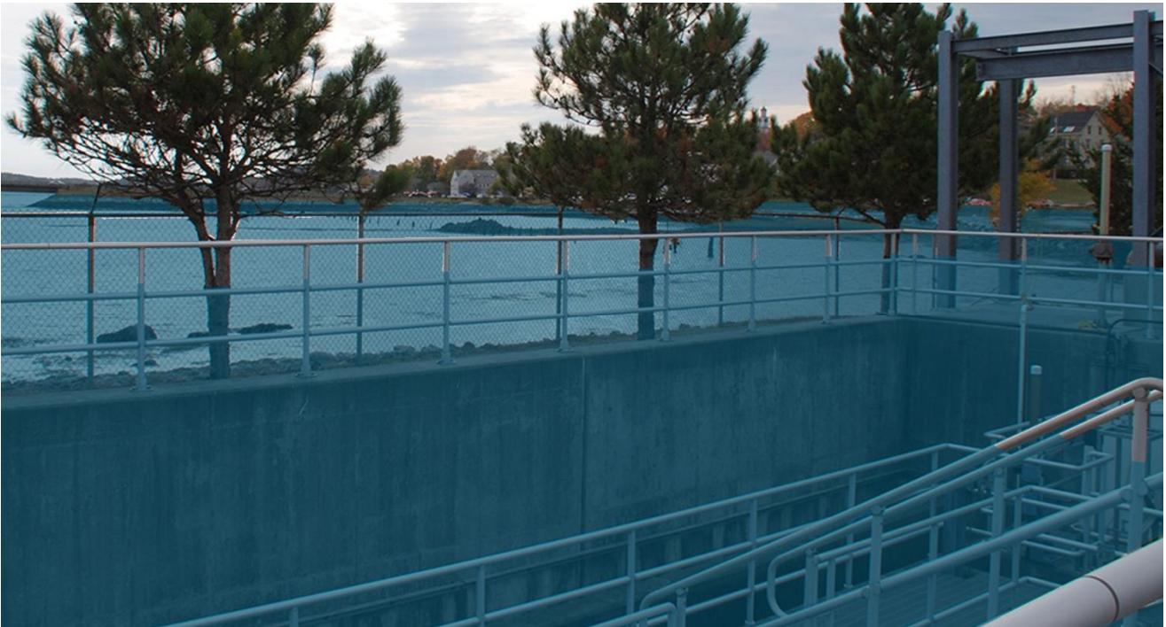
Chlorine Contact Tank Looking South – BFE +4
