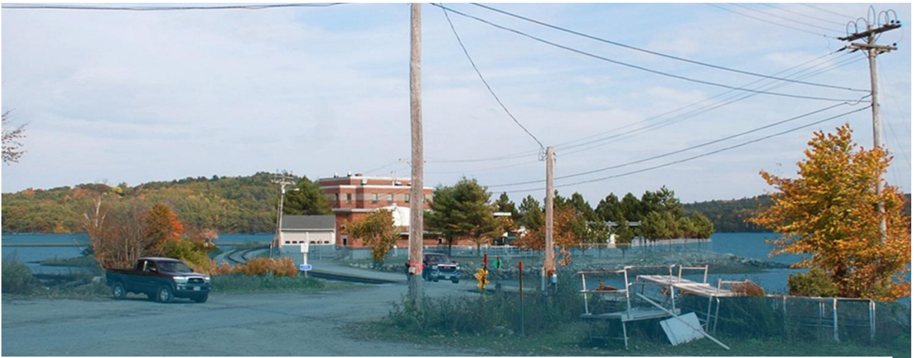
Site Approach Along Railroad Avenue Looking North Towards The WWTP – BFE +3
