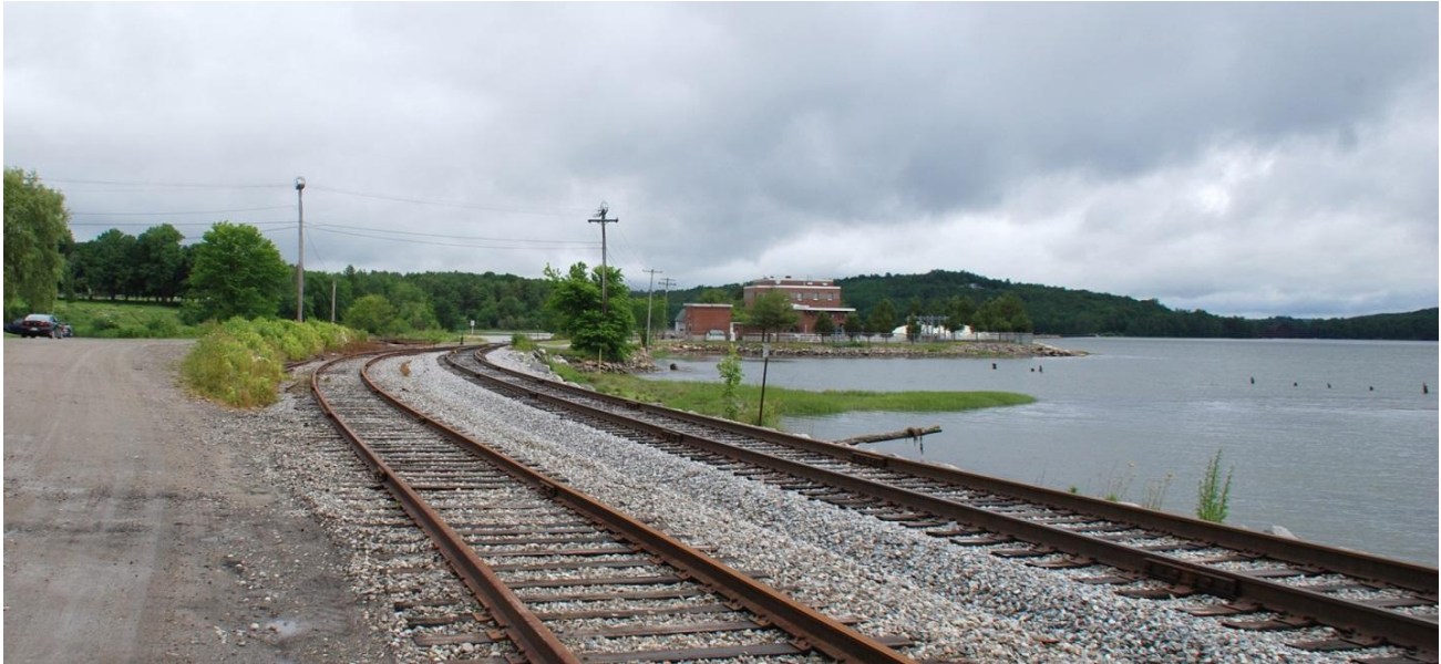
View of WWTP from Railroad Avenue and the Maine Central Railroad
