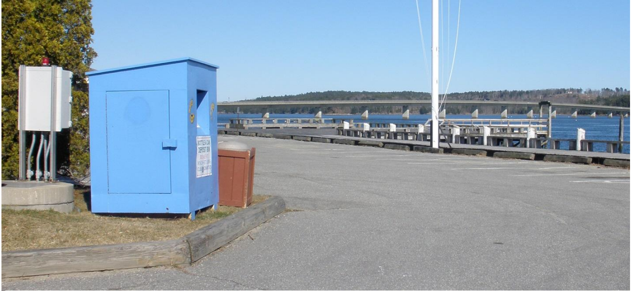
Water Street Pump Station on the far left with the Recreational Pier in the background
