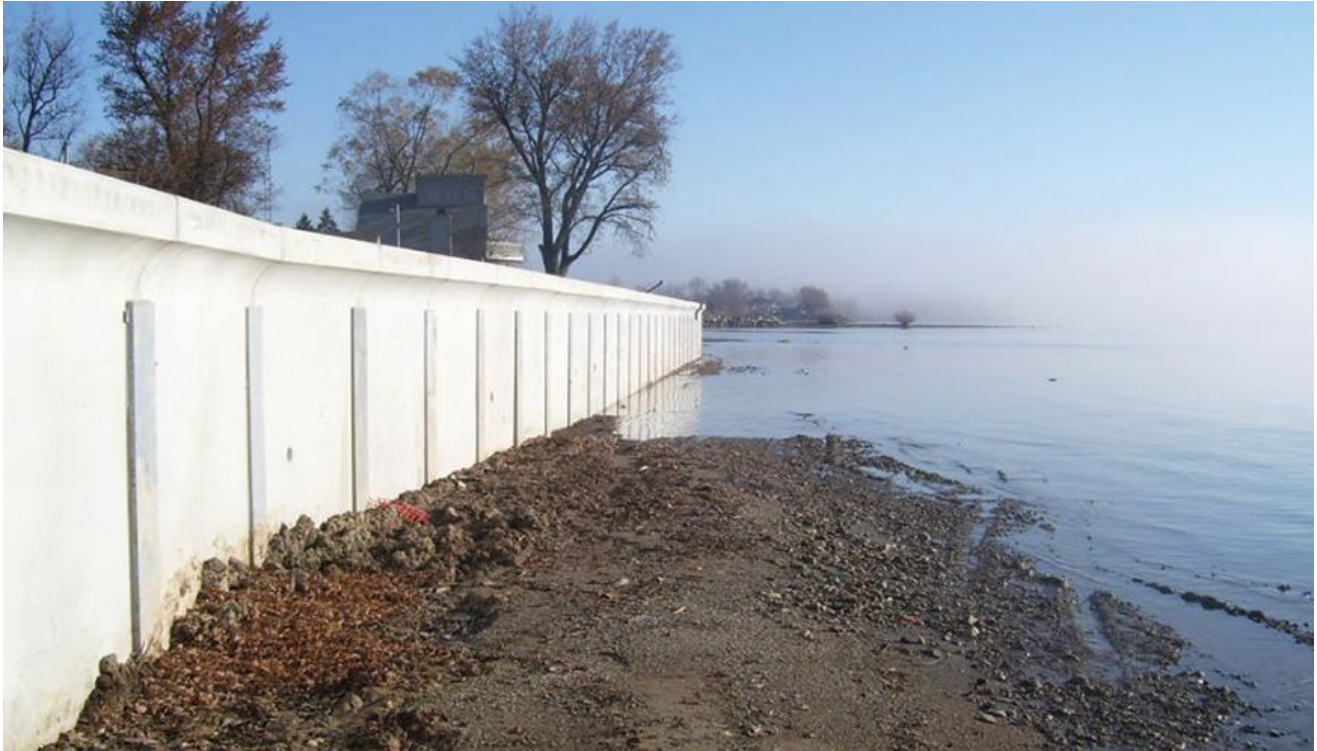
Example of a concrete barrier sea wall (Source from Ohio Department of Natural Resources Office of Coastal Management)
