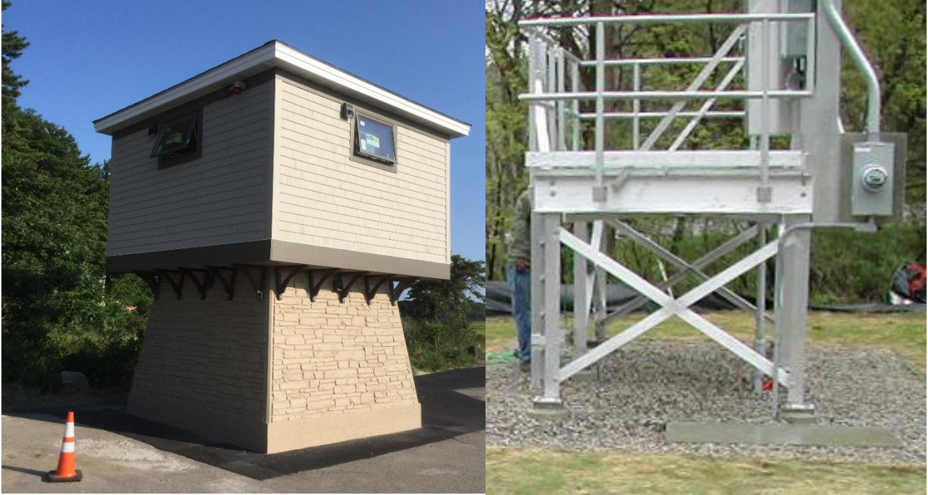
Examples of elevated structures to house electrical supply and controls systems, as well as emergency power generator and fuel storage. Ogunquit, ME on left. Skowhegan, ME on right
