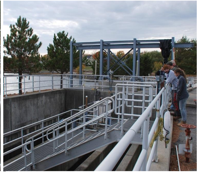
Chlorine contact tank
