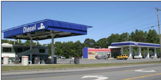
Figure 2-31 A well maintained, but highly visible gas station
