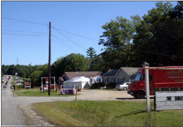
Figure 2-24 Strip development – expansive and cluttered views
