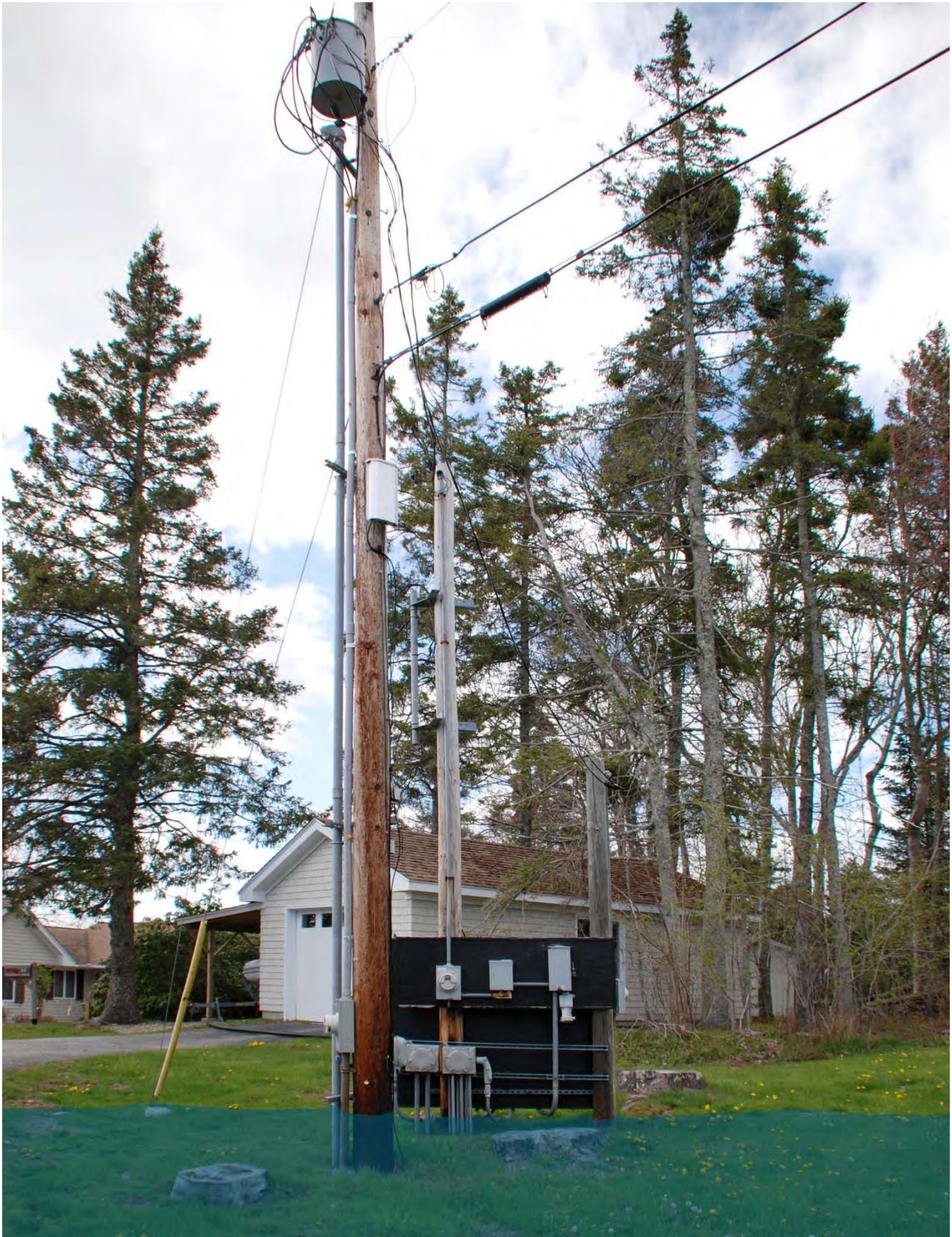
PS #13 Electrical Service and Controls - BFE +6
