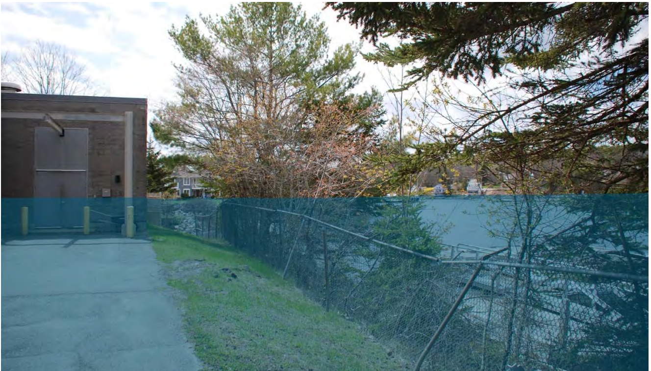
WWTP Looking West at Process Building and Boothbay Harbor - BFE +5
