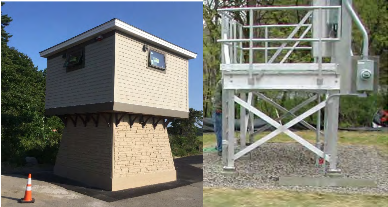
Examples of Elevated Structures to House Electrical and Control Panel Systems, as well as Emergency Power Generators from Other Maine Communities
