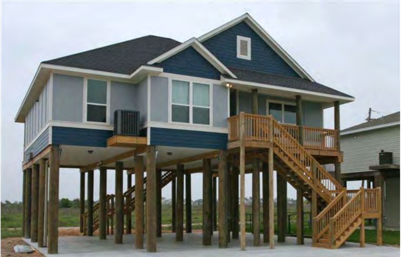
Example of Building Elevated on Pile Supports (source from internet)
