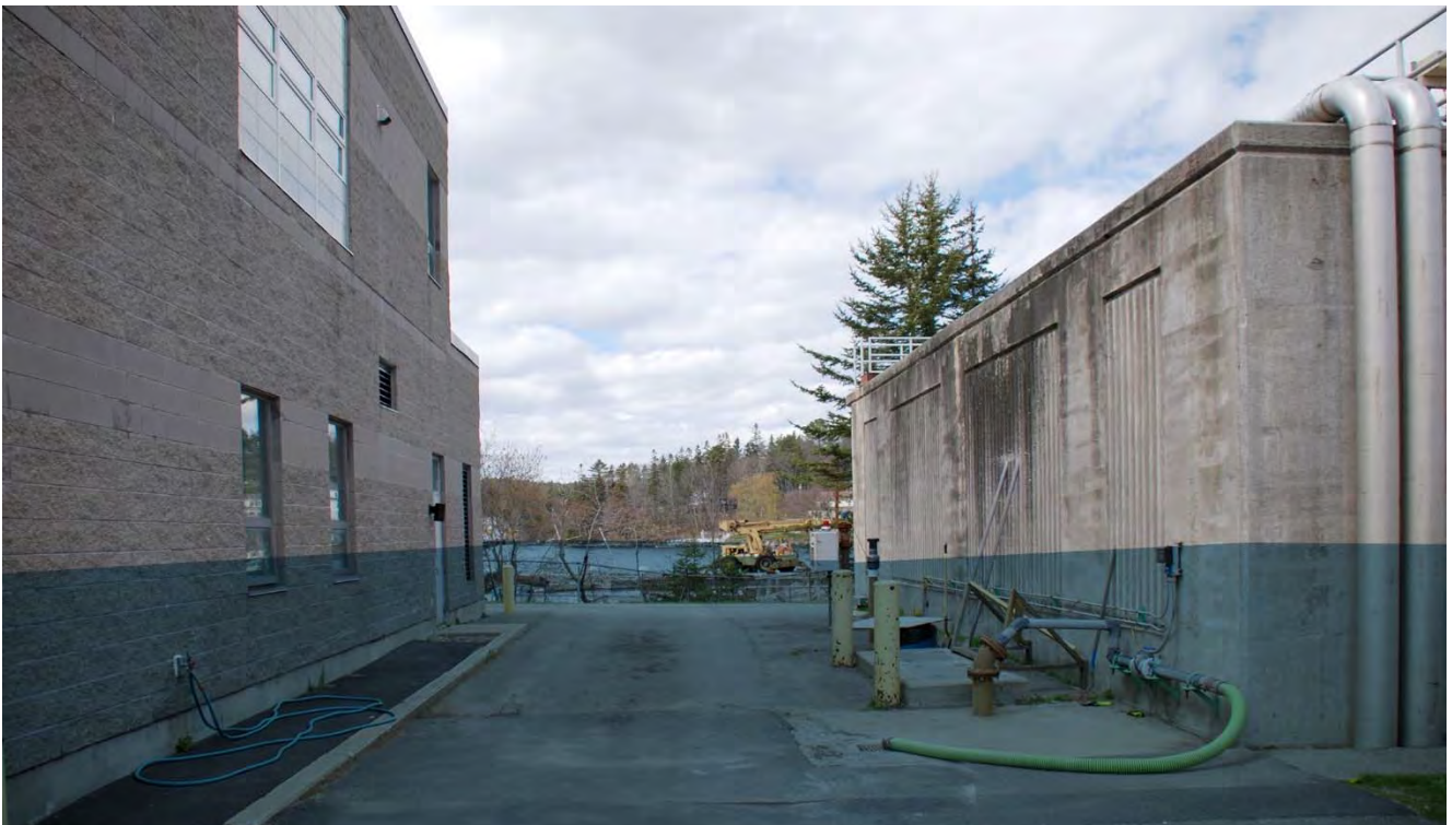
WWTP Looking North Between the Process Building and SBRs – BFE +5
