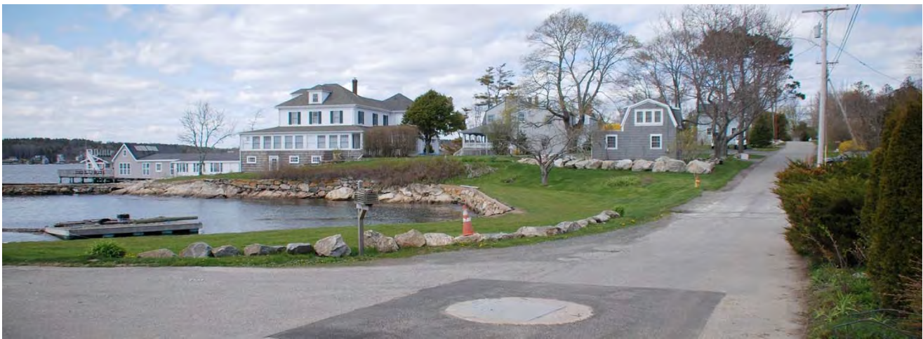
PS #12 Wetwell Looking East Along Roads End Road
