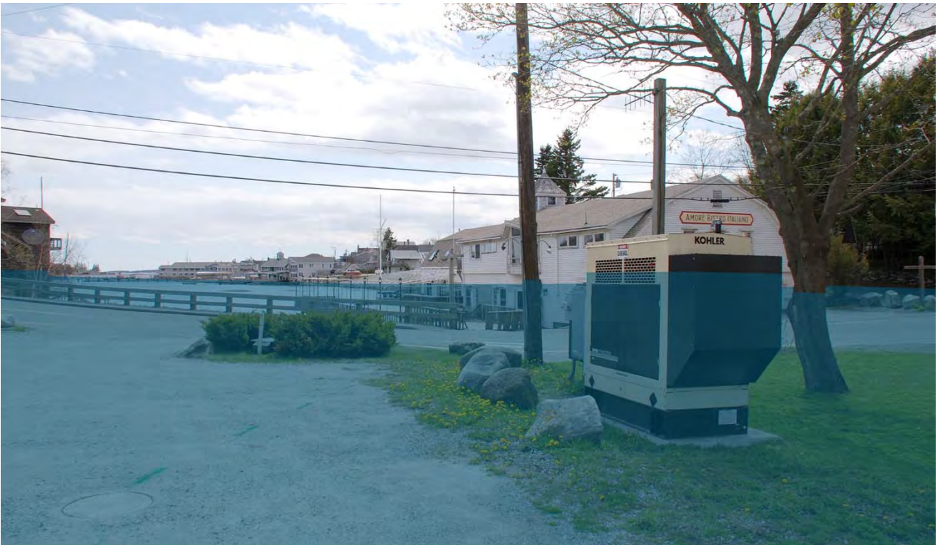
PS #1 Looking West Across Union Street and Towards Boothbay Harbor - BFE +5
