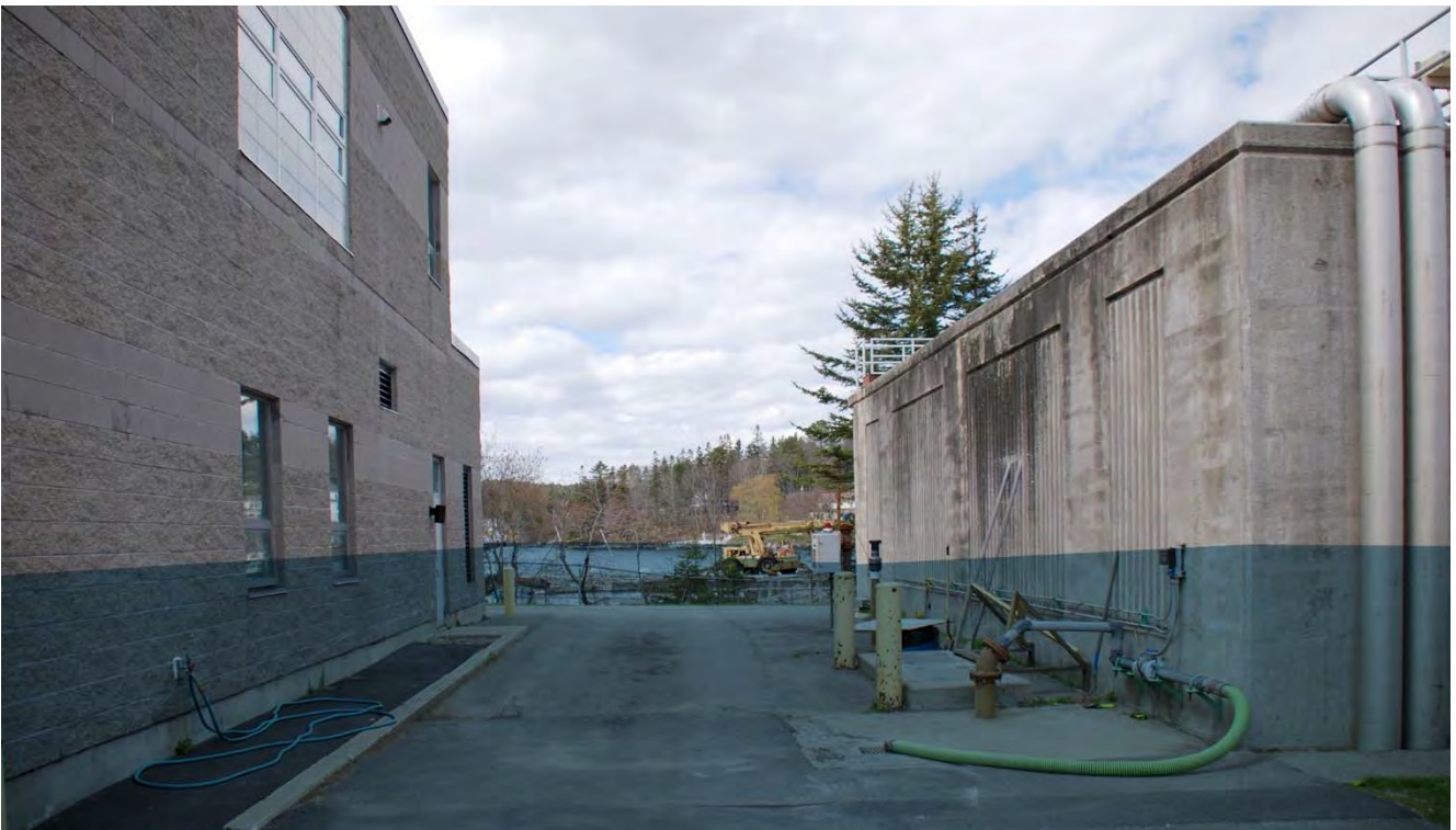
WWTP Looking North Between the Process Building and SBRs – BFE +6
