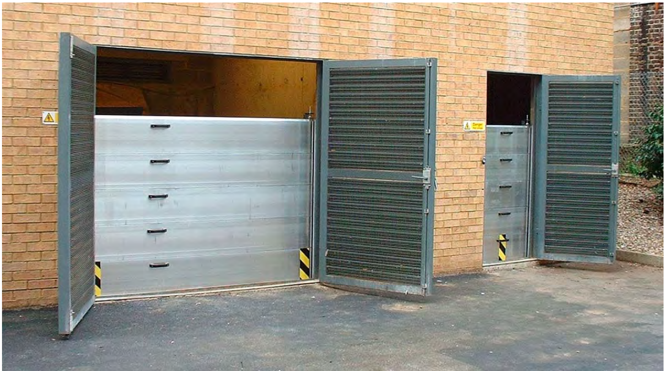
Examples of Temporary Flood Barriers for Doors (source from internet)
