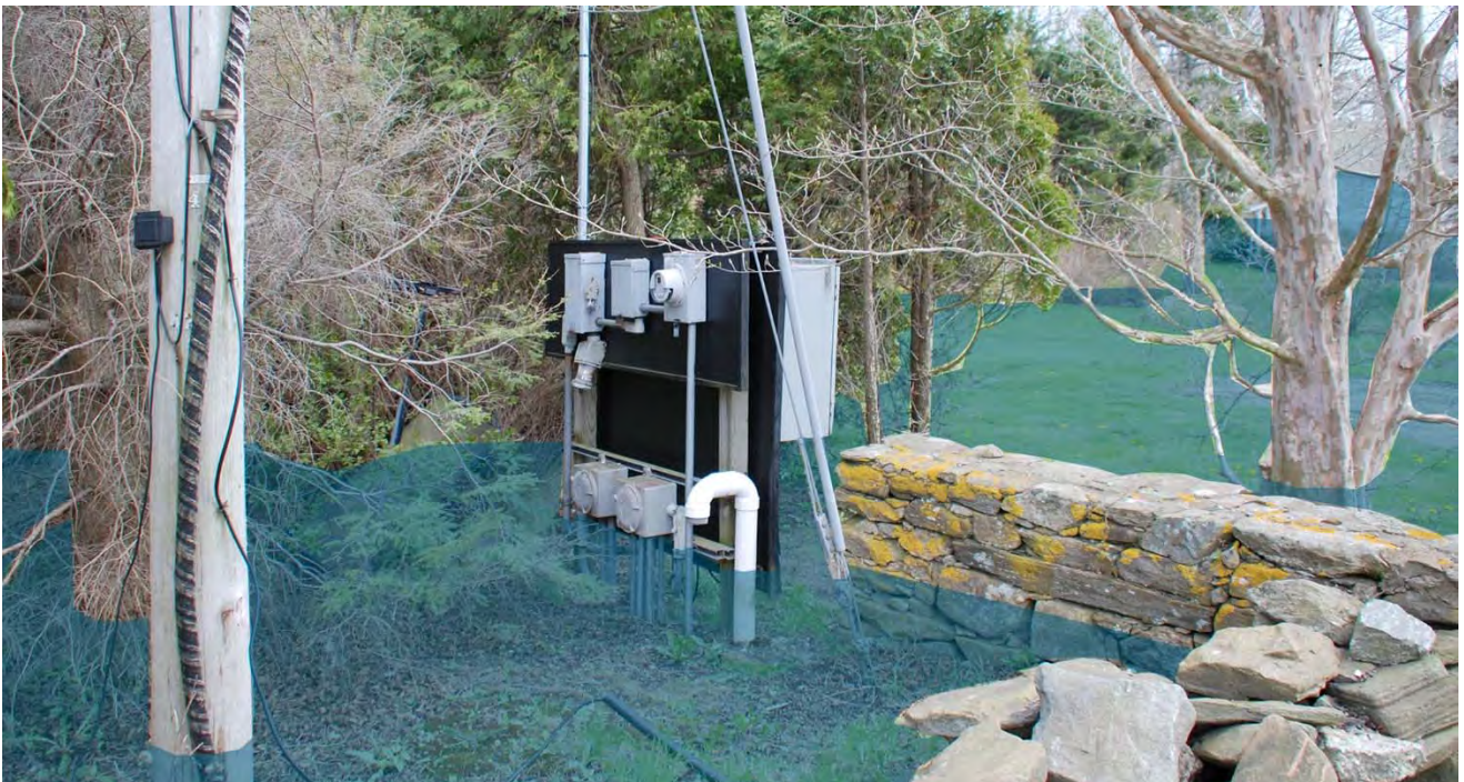
PS #12 Electrical / Controls Panel Looking South - BFE +4
