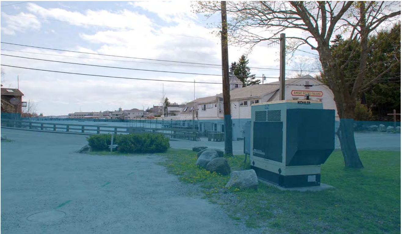
PS #1 Looking West Across Union Street and Towards Boothbay Harbor - BFE +6
