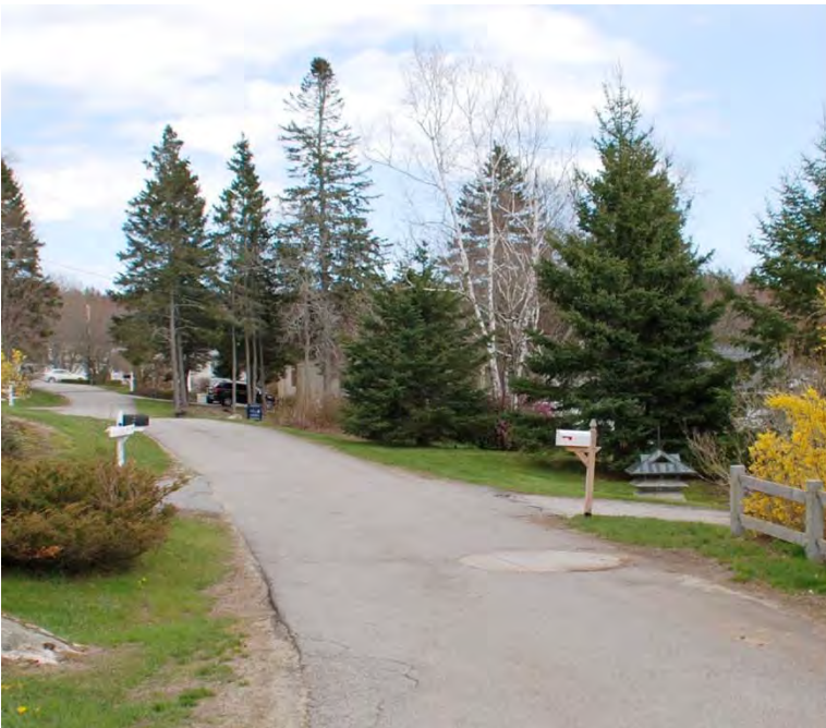
PS #13 Wetwell Looking East Along Factory Cove Road
