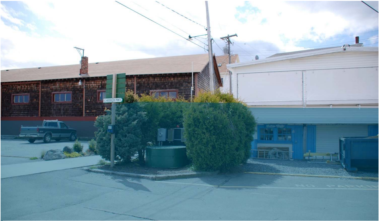
PS #7 Looking North Towards Townsend Avenue from Boothbay Harbor - BFE +5
