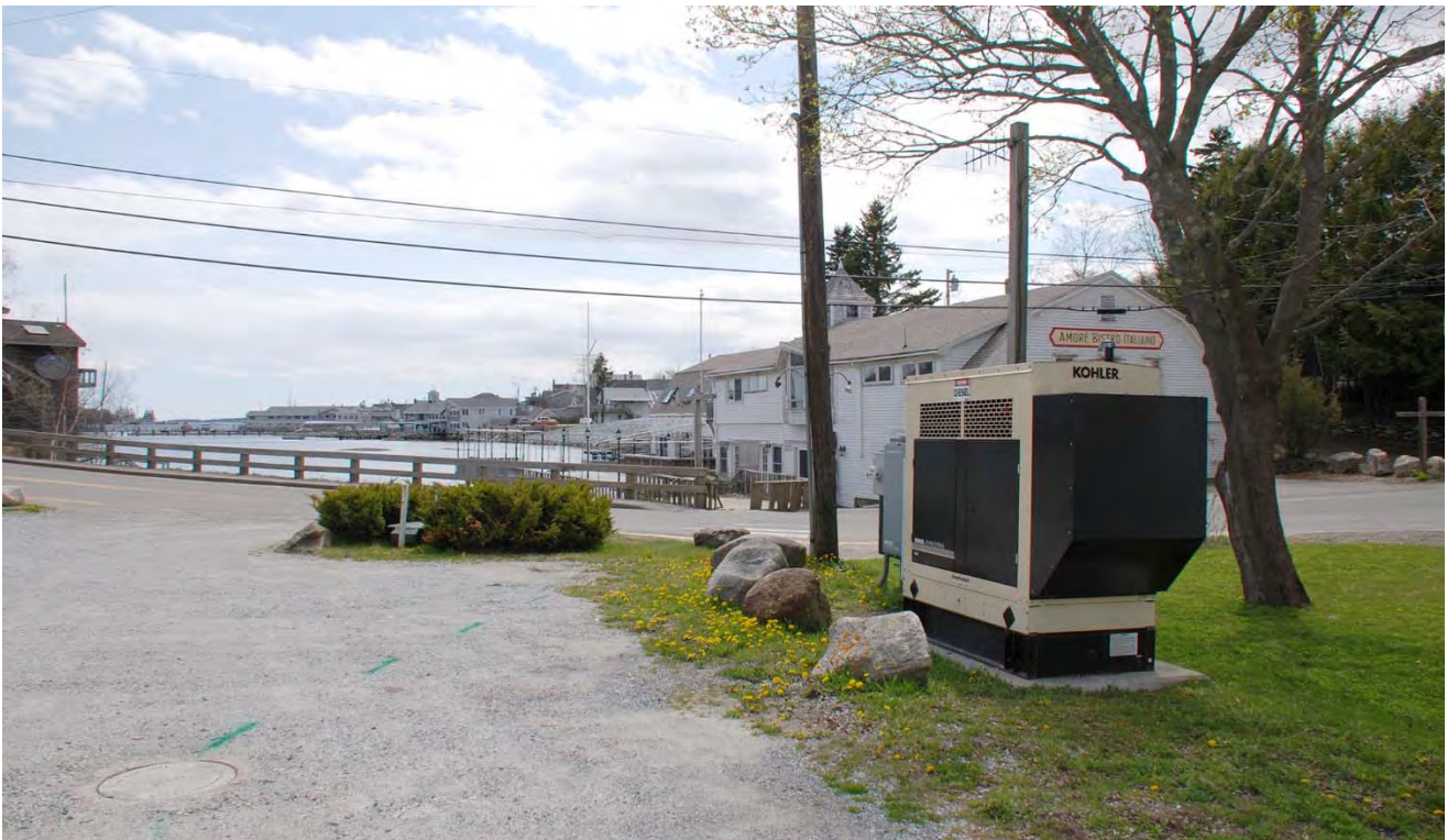
PS #1 Looking Across Union Street Towards Boothbay Harbor
