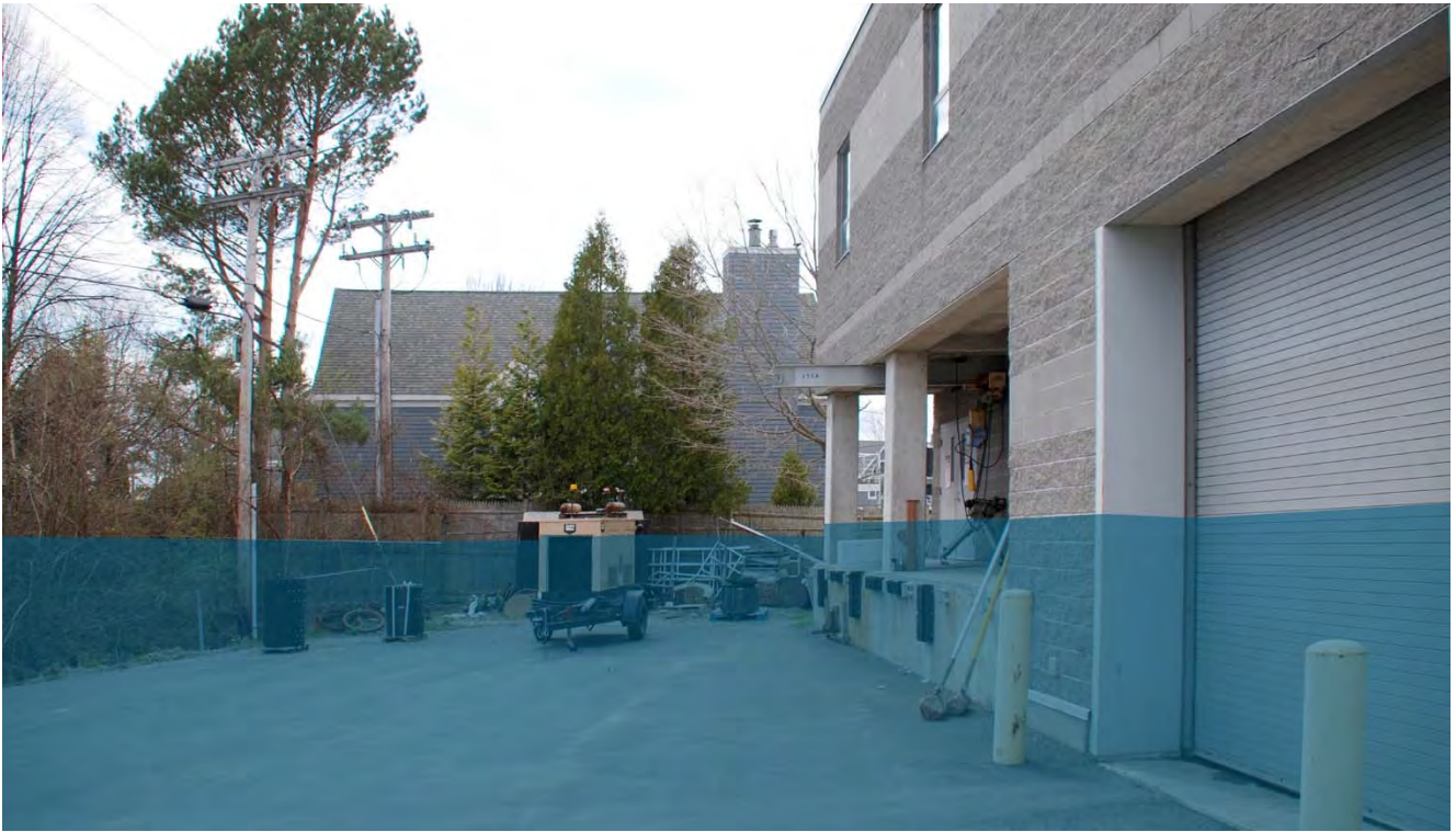
WWTP Looking West Past the Process Building - BFE + 6
