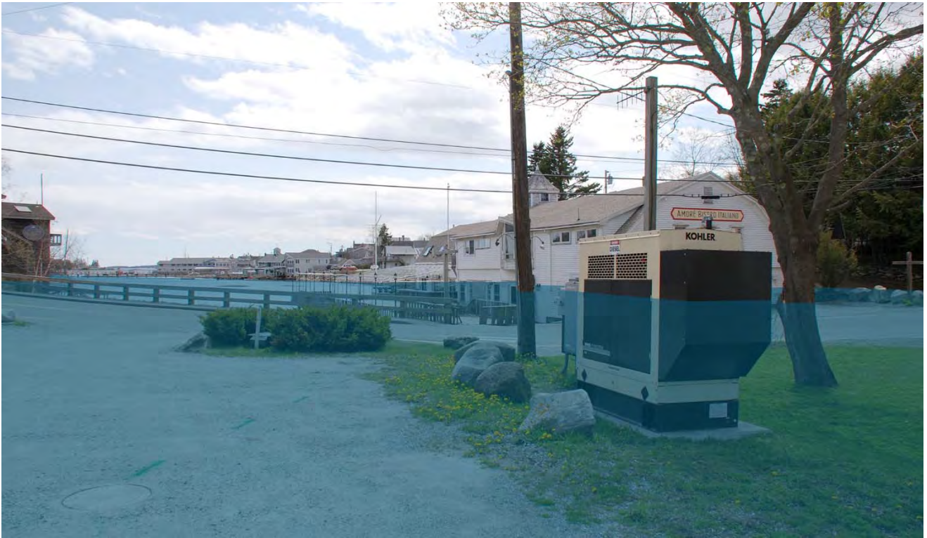
PS #1 Looking West Across Union Street and Towards Boothbay Harbor - BFE +4
