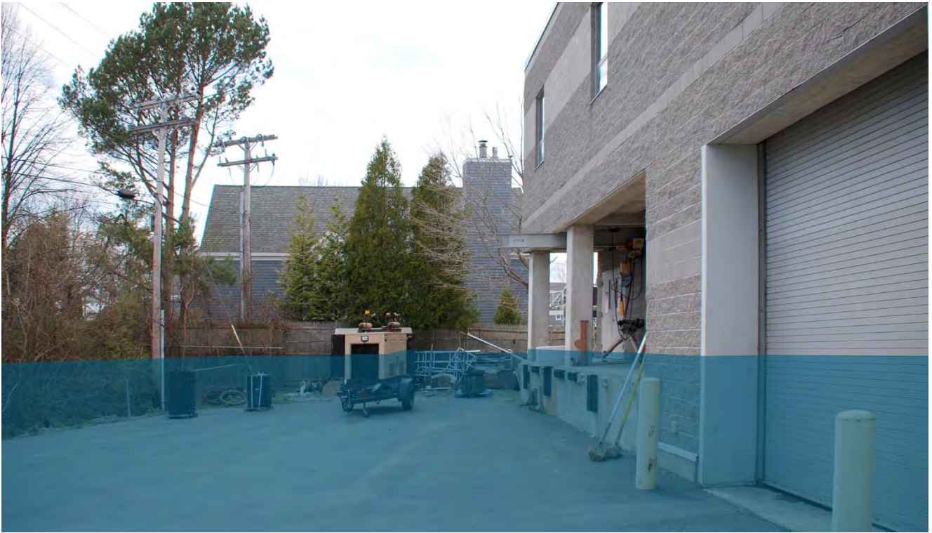
WWTP Looking West Past the Process Building - BFE +5
