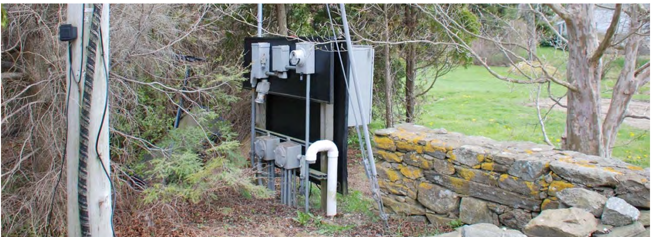
PS #12 Controls West Towards Boothbay Harbor
