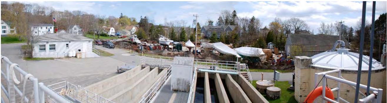
View of the WWTF Looking South from the top of the Sequencing Batch Reactors
