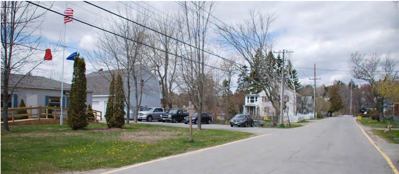
Sea Street Looking North from the WWTF Entrance. Admin. Building and Garage on the Left
