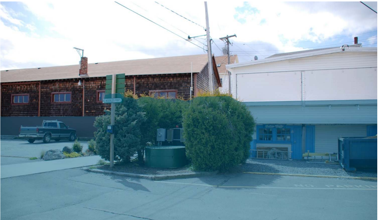
PS #7 Looking North Towards Townsend Avenue from Boothbay Harbor - BFE +6
