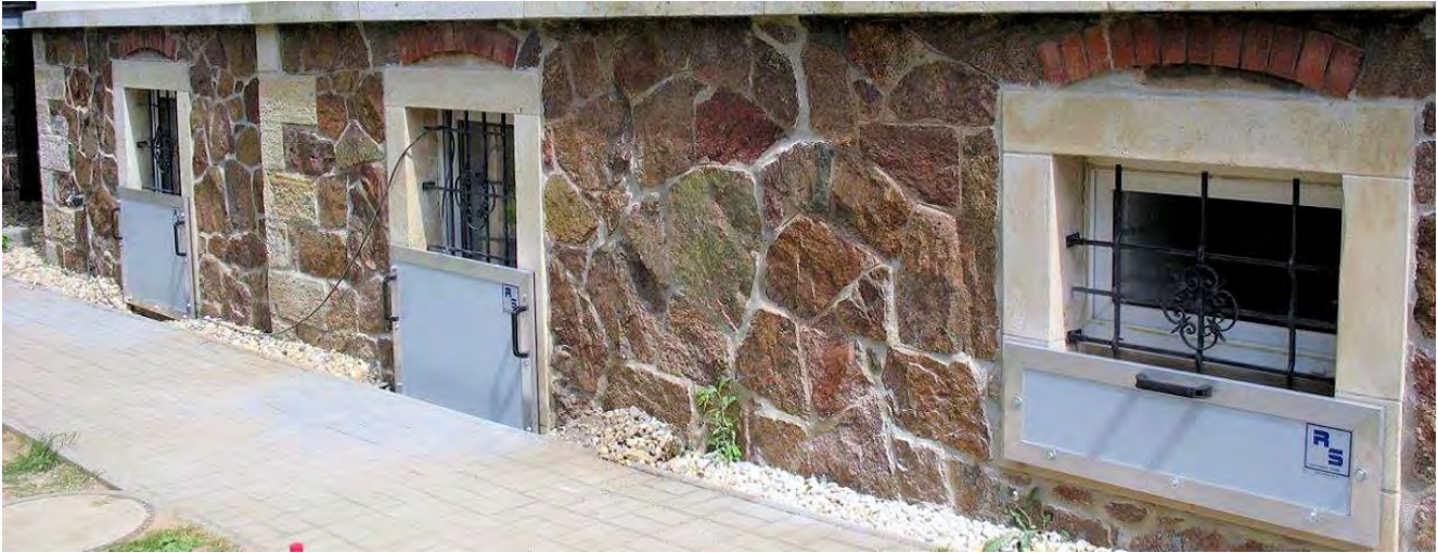
Examples of Temporary Flood Barriers for Windows (source from internet)
