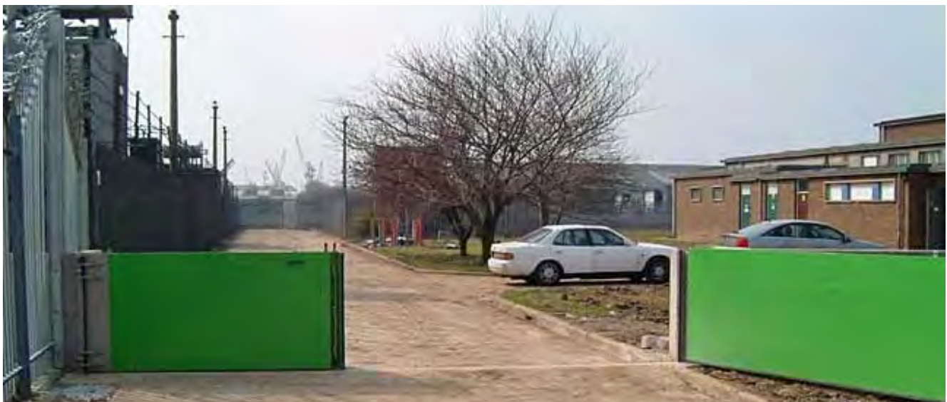
Example of a Barrier Wall and Flood Gates (sources from internet)
