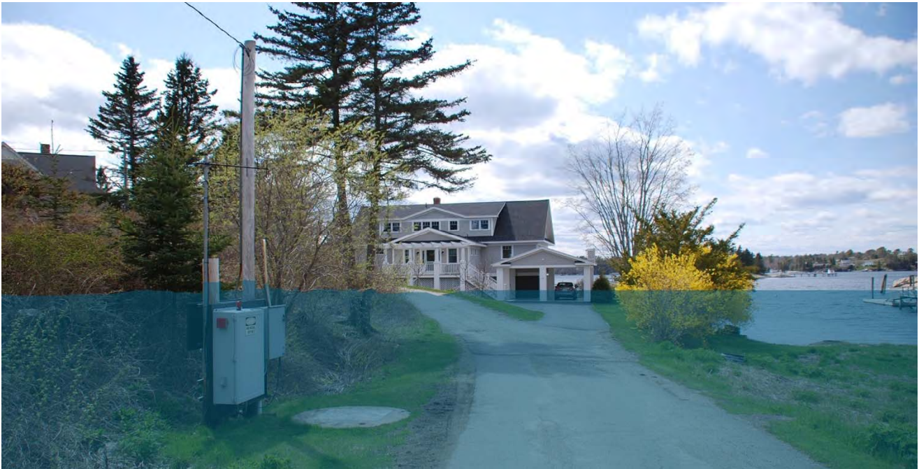
PS #15 Looking West Towards Boothbay Harbor - BFE +6
