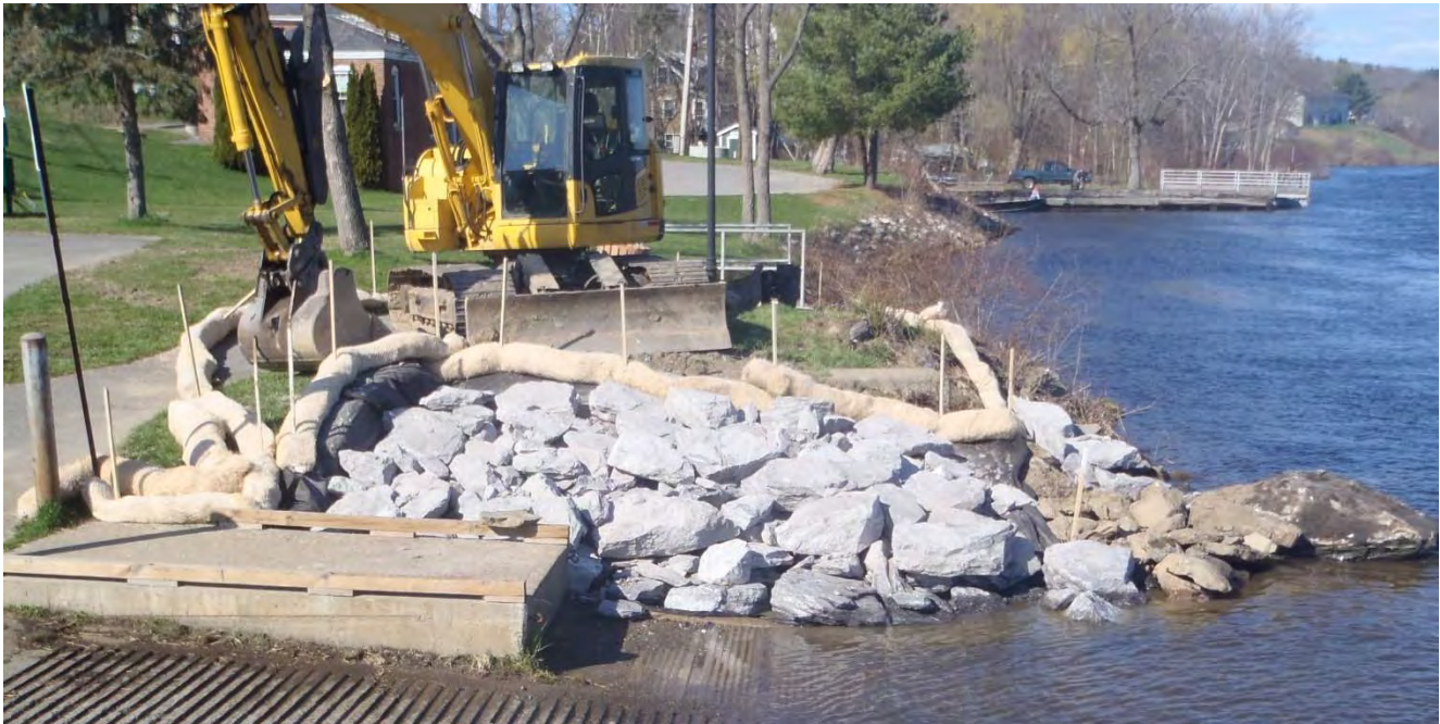
Examples of Heavy Riprap Shoreline Stabilization in Richmond, Maine
