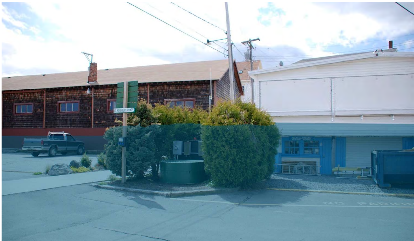
PS #7 Looking North Towards Townsend Avenue from Boothbay Harbor - BFE +4
