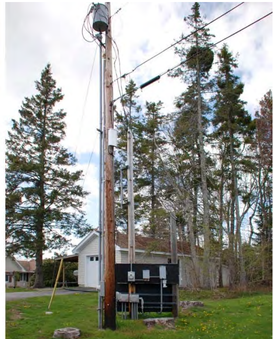
PS #13 Controls Looking East
