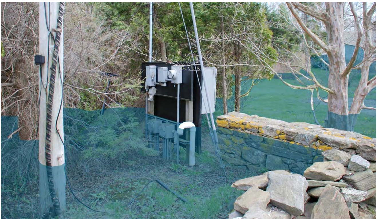
PS #12 Electrical / Control Panels Looking South - BFE +5
