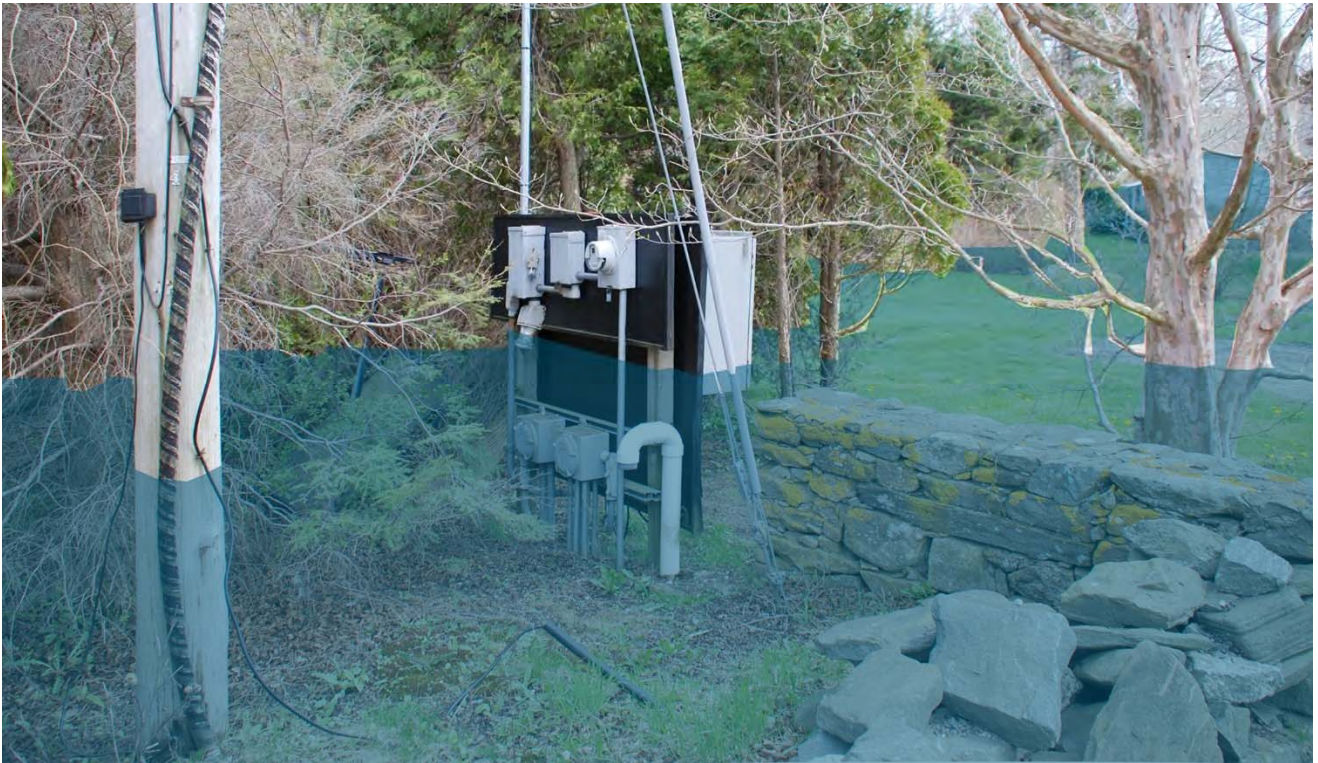
PS #12 Electrical / Control Panels Looking South - BFE +6
