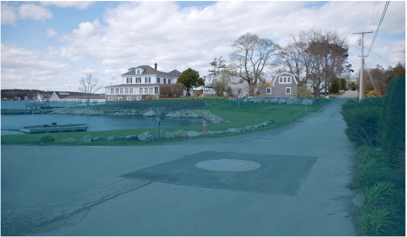
PS #12 Wetwell Looking North - BFE +6
