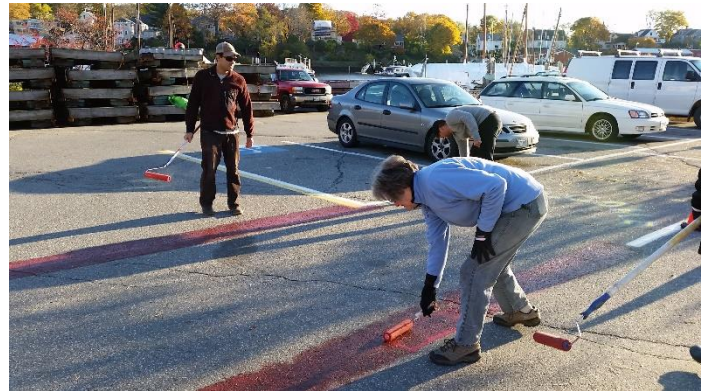
Figure 29: Painting new red walkways with temporary chalk paint
