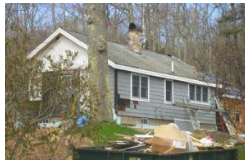
Camden Single Family Housing Rehabilitation
