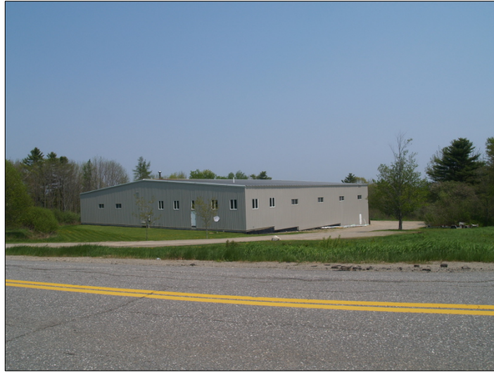
Building fully exposed to view.
