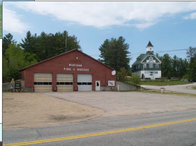
Recent construction that is incompatible in style, color, shape and mass with nearby historic building.
