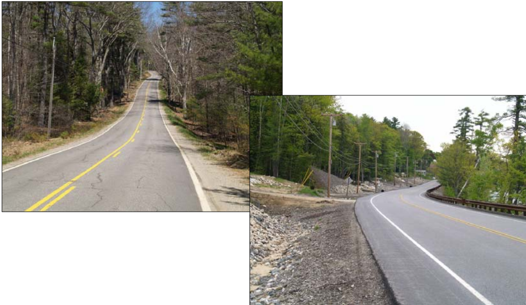
Formerly rural road with extensive clearing and re-grading.
