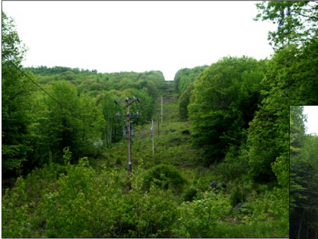
Utility corridor perpendicular to view from road.
