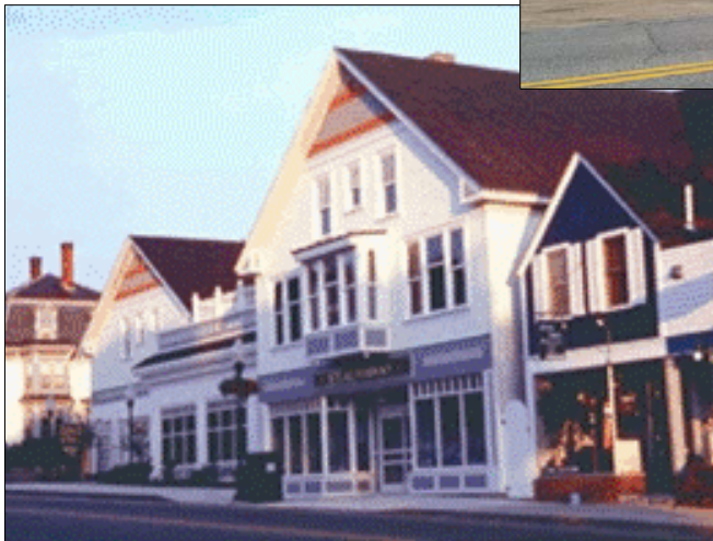
Traditional facades in village center.
