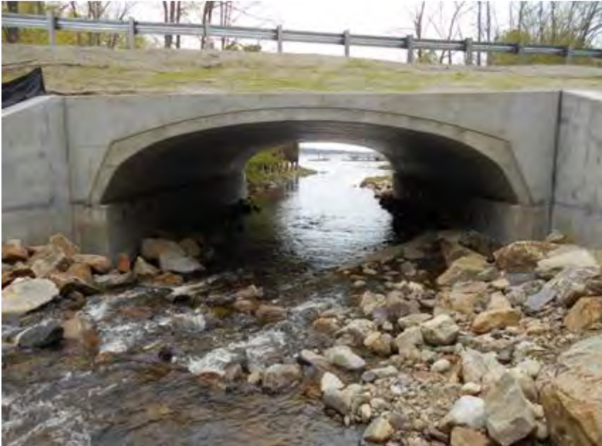
Figure 14.14 Tidal Crossing Box Culvert Structure Installed in Northport
