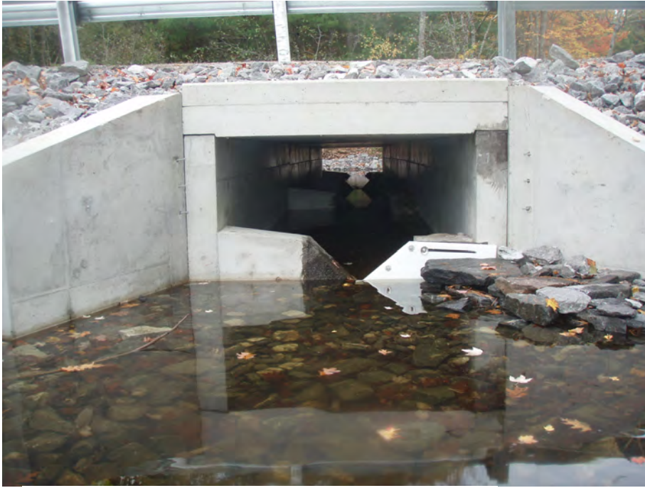
Figure 6.7 Box Culvert at Sewell Pond in Arrowsic
