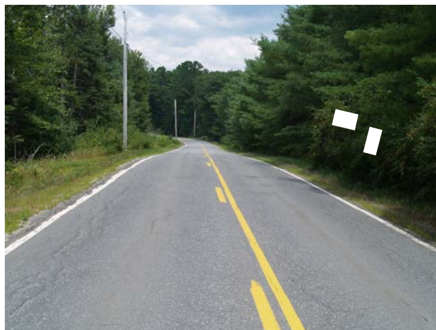
Figure 6 Manktown Road in Vicinity of Public School Complex
