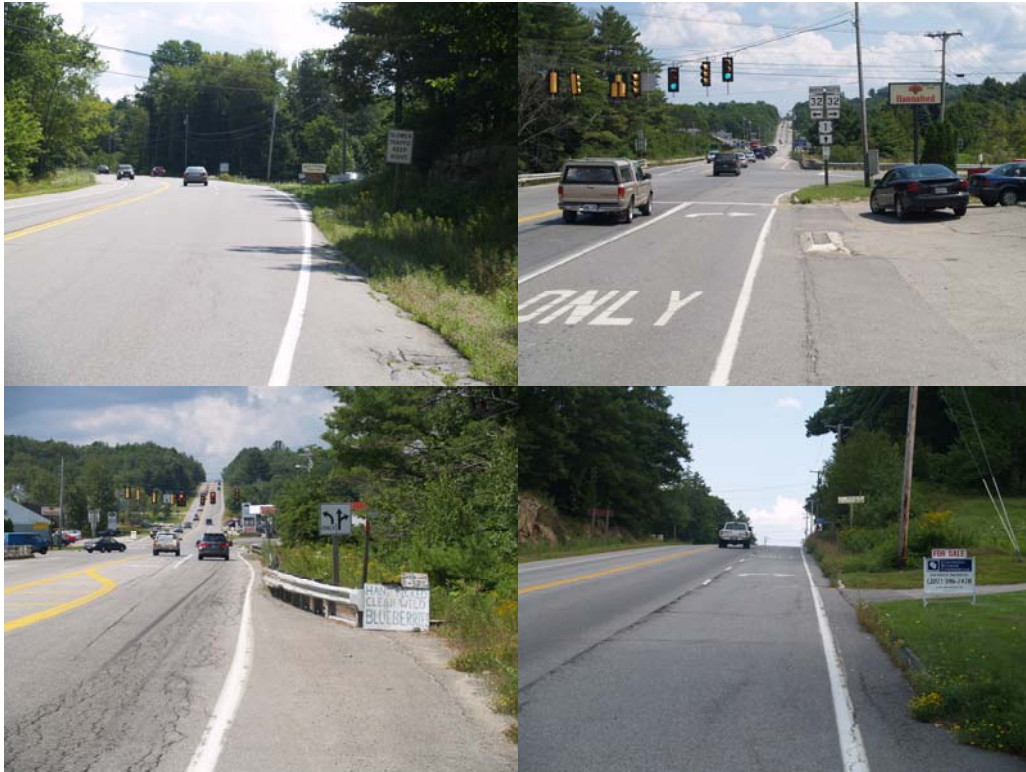
Figure 12 Route 1 Paved Shoulders
