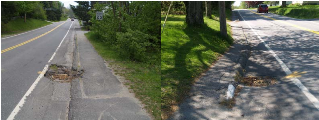
Figure 11 Depressed Grates on Friendship Road and Bremen Road
