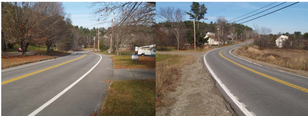
Figure 6 Route 218/Federal Street
